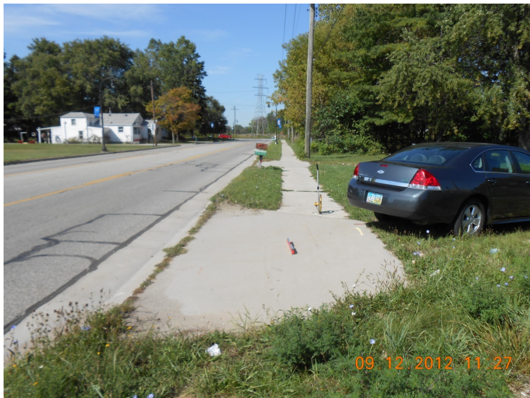
Picture 3: Start of existing sidewalk on Howard, looking west.
