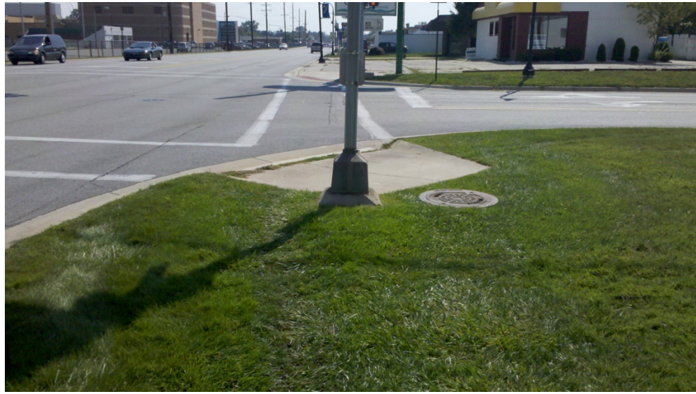
Picture 6: Isolated crosswalk ramp at Howard Street and 24 th Street, looking south.
