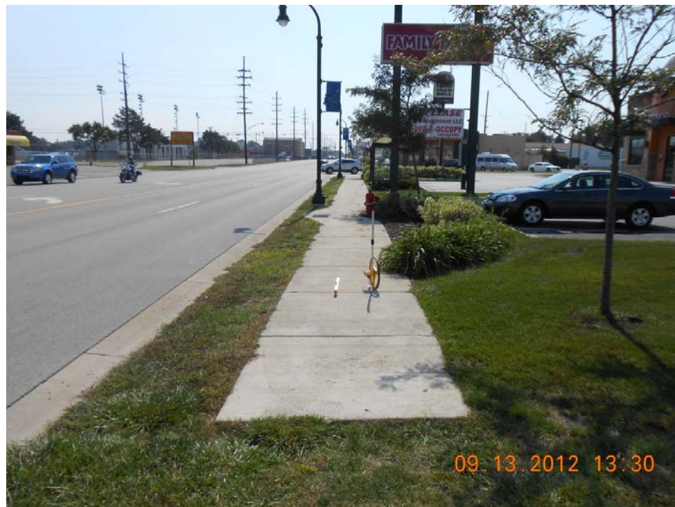
Picture 4: Start of existing sidewalk on 24th Street, looking south.
